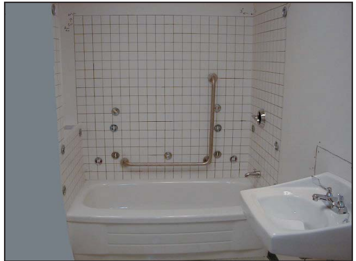
Figure 3 : Ontario Building Code (OBC) modified configuration
